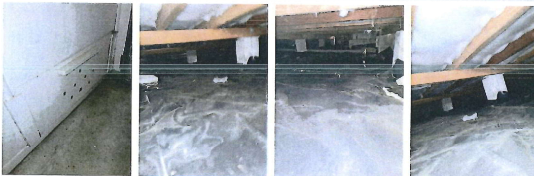
On-Ground Vapour Barrier Photos
