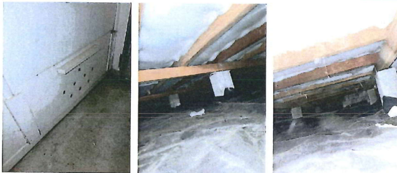
Underfloor Insulation Photos
